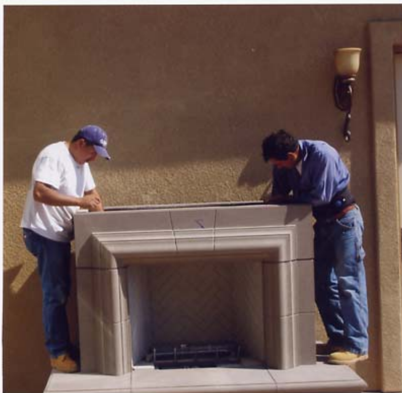
Stack and bolt subsequent sections
