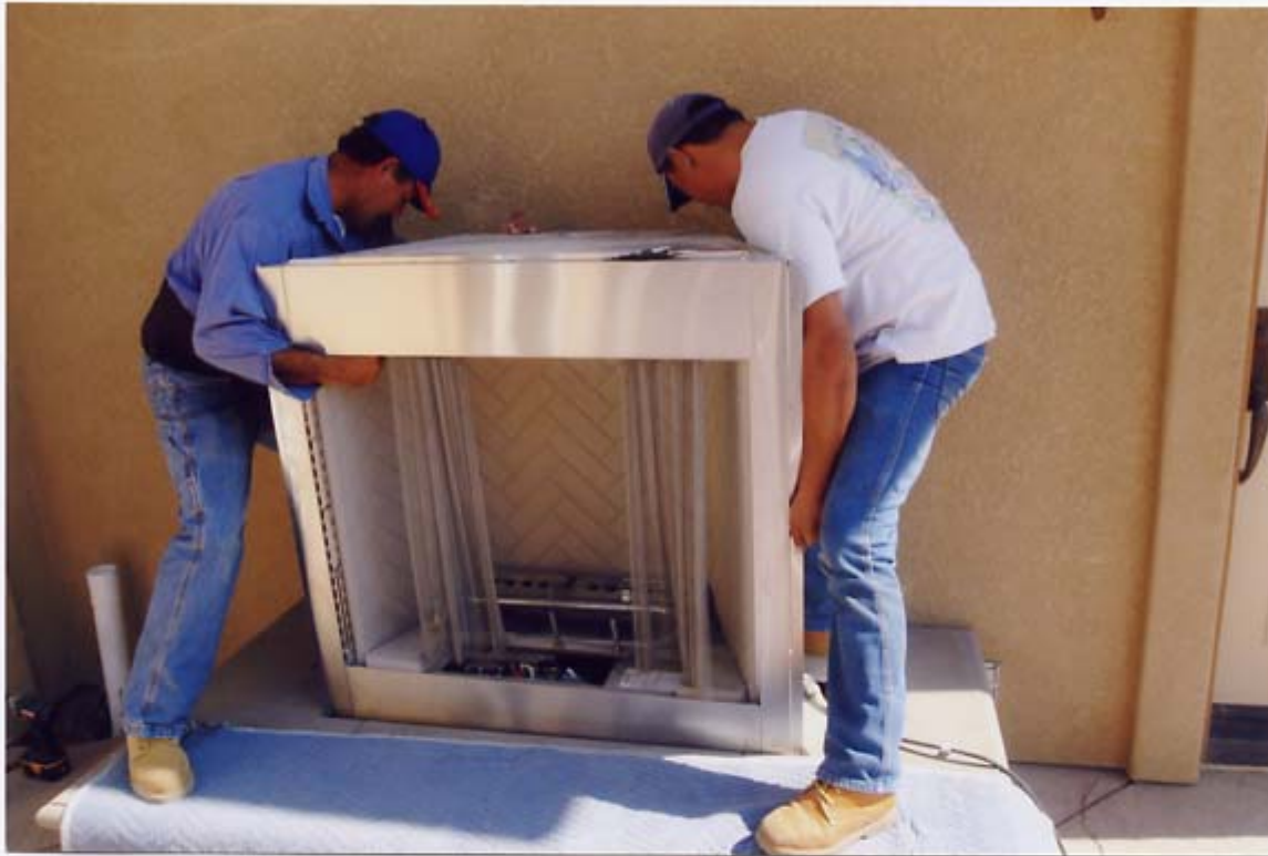
With hearth in place, install firebox
