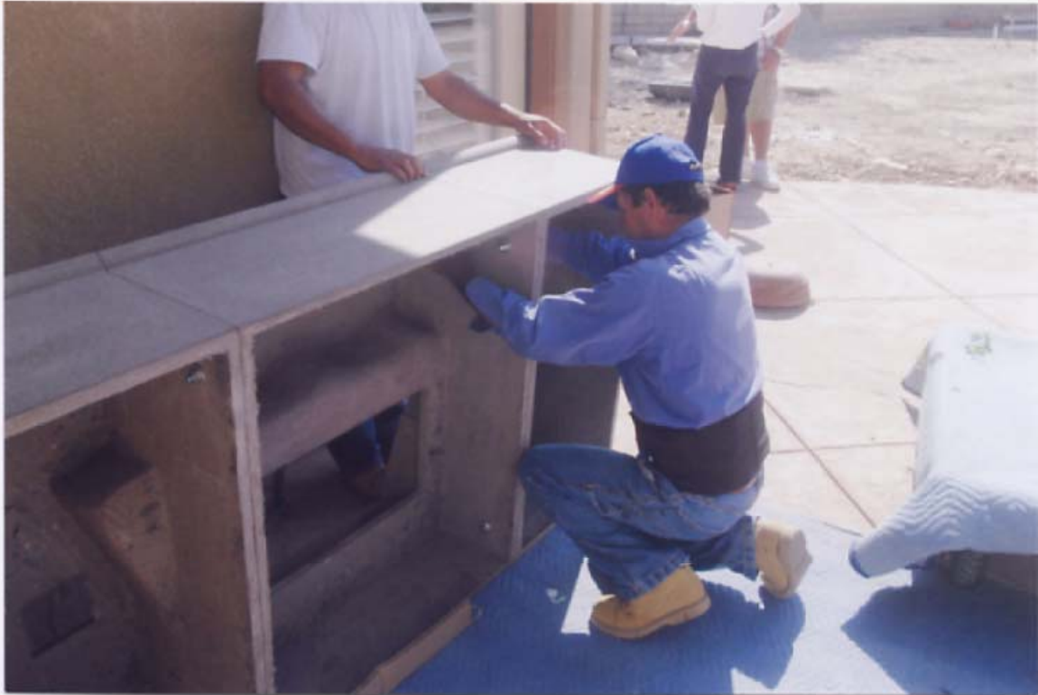
With hearth tilted on back, bolt together
