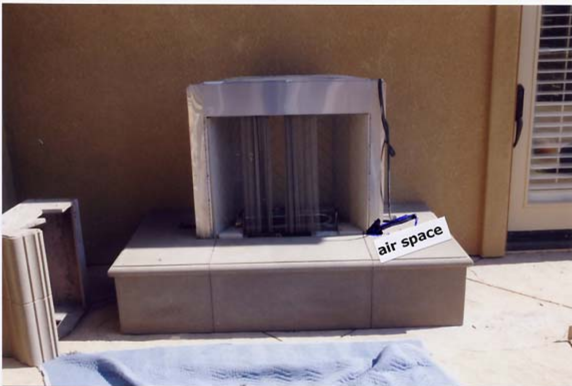
With firebox in place, now is the time to make ALL GAS connections . Make sure there is air space between front of firebox & hearth for ventilation
