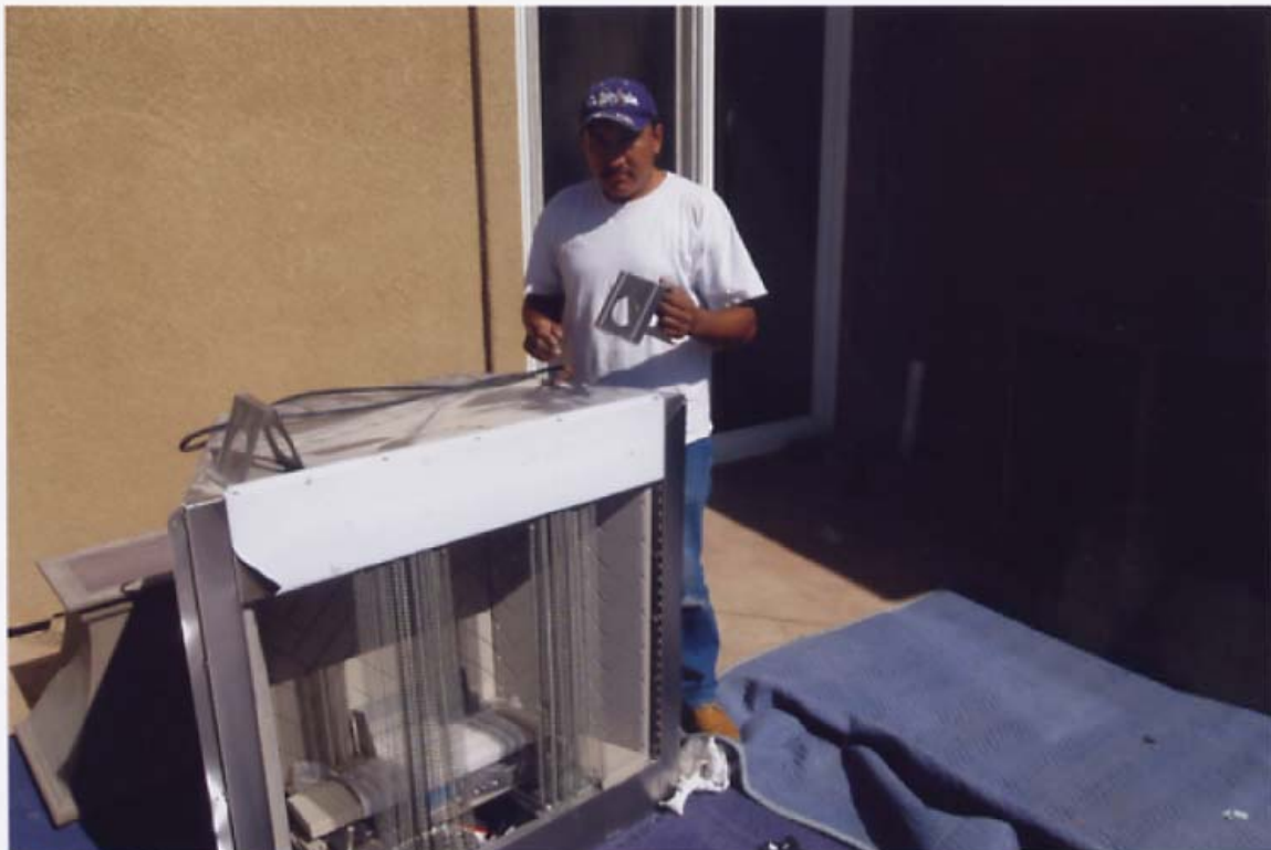
Remove protective pieces from Ventless firebox
